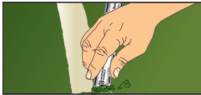
Remove turf with Road Scraper.
